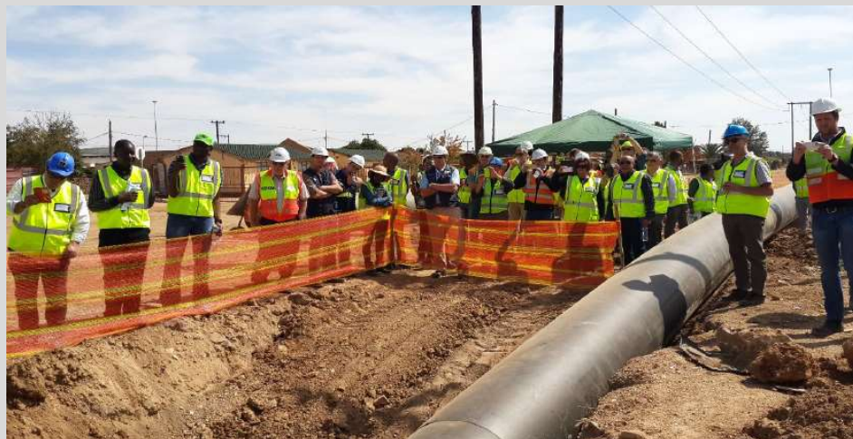
Polyethylene water pipe being installed outside Hammanskraal ( Material and images courtesy of Trenchless Technologies )
